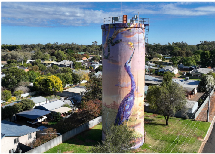
20. Hillston Water Tower. Artists Down Under (2012)
