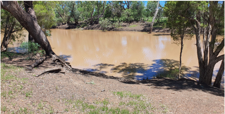
Figure 027. - Exposed and eroded riverbanks (McGregor Coxall).
