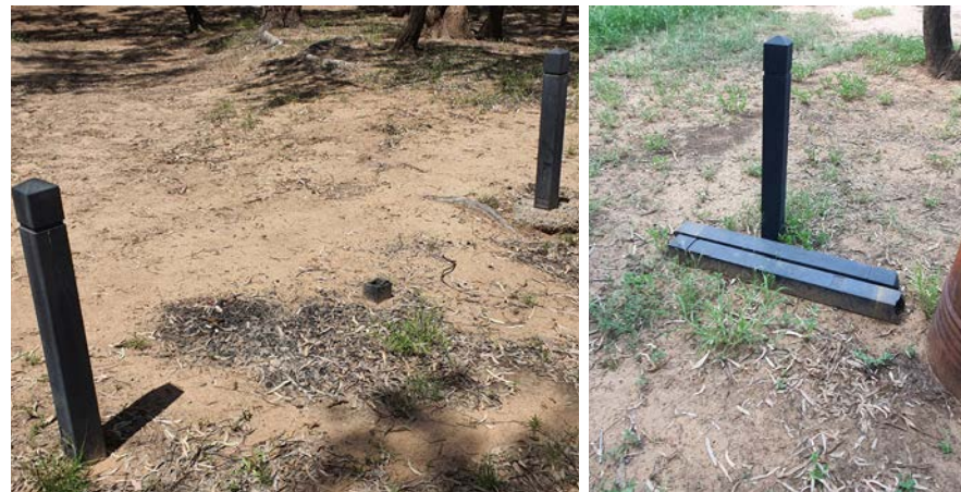
Figure 032. - Vandalised bollards intentionally removed by vandals to gain unauthorised access to the riverbank (Images by McGregor Coxall).
