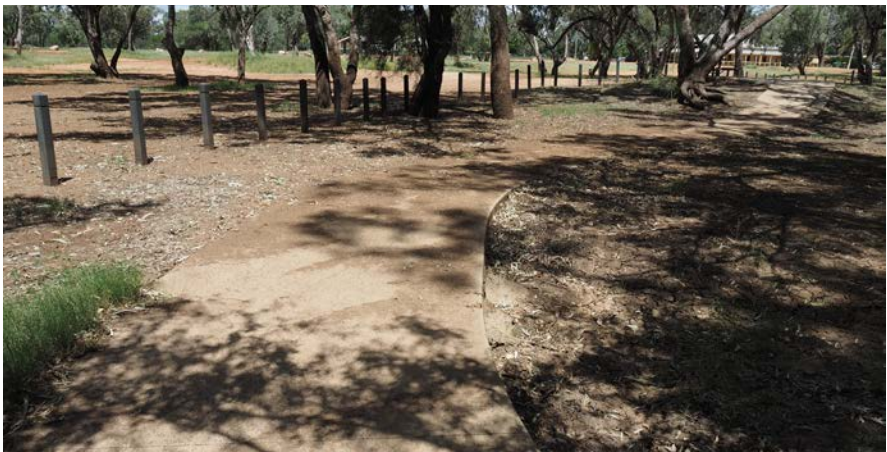
Figure 025. - Low lying existing footpath covered in silt from recent overland flow of rainfall and/or flooding (Image by Rounsefell Design).
