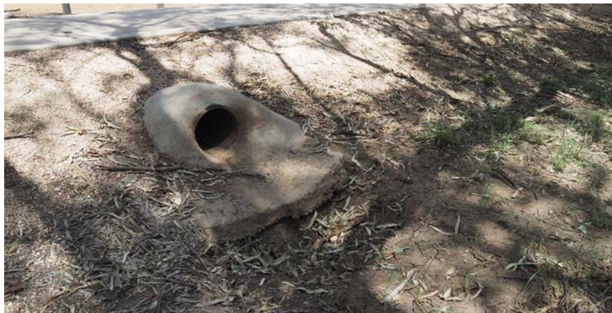
Figure 031. - Insufficient stormwater piping beneath raised pathways causing flow issues and creating localised outfall erosion issues (Image by Rounsefell Design).
