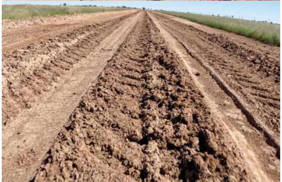
Two separate roads showing damage caused by trucks driven over a saturated surface.
