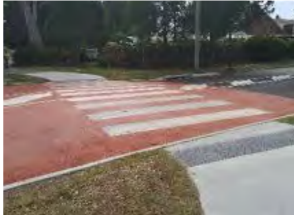
Decorative Road Surfacing
