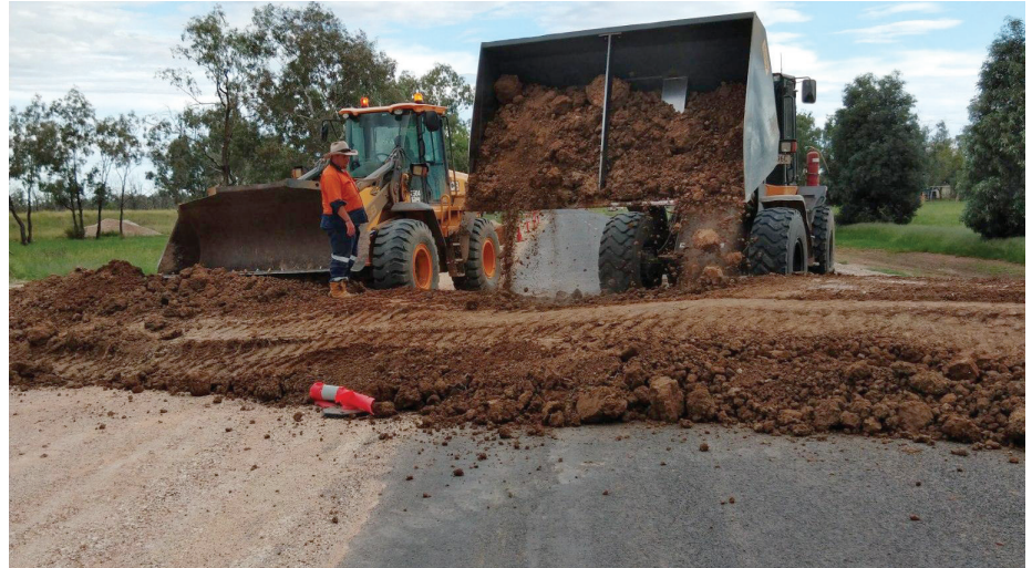
Balonne Shire Council staff closing the levee at Thallon.
