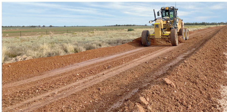
Work on Gunnindaddy Road.
